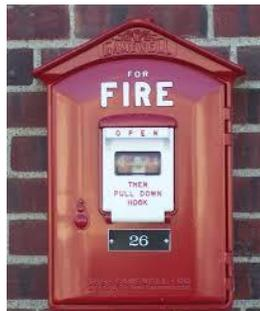
The Gamewell fire alarm system was put into use in the early 1880's. This system was distributed throughout the city for the citizens to contact the fire department. This system remained in place until February 1, 1994 when the duties of the municipal alarm system, (or box alarm system) were relinquished to outside alarm contractors under control of the county government.
